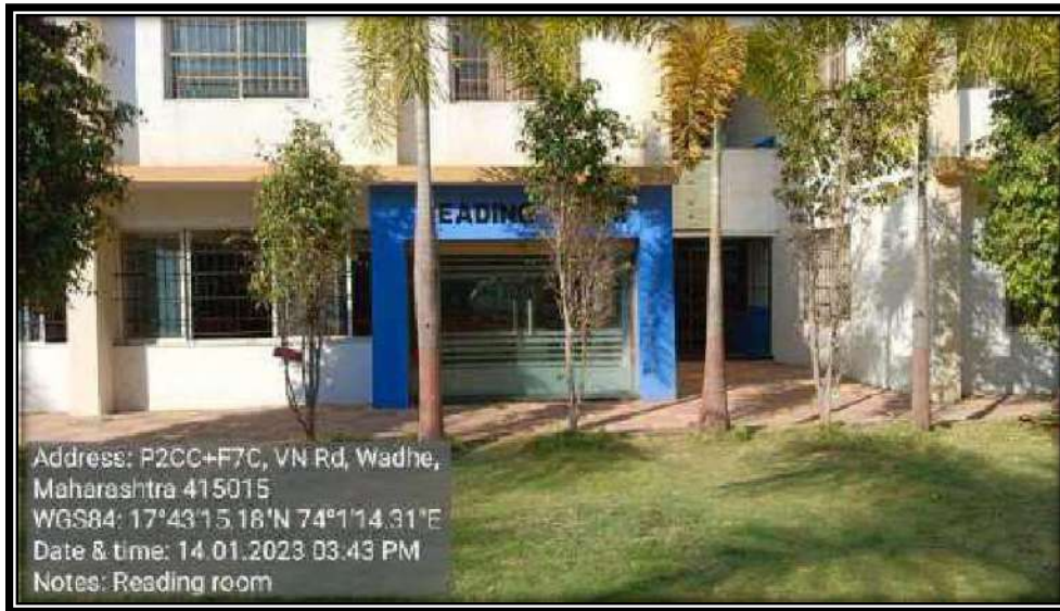
Fig. 7.1.3.2. Landscaping in the YTC campus
